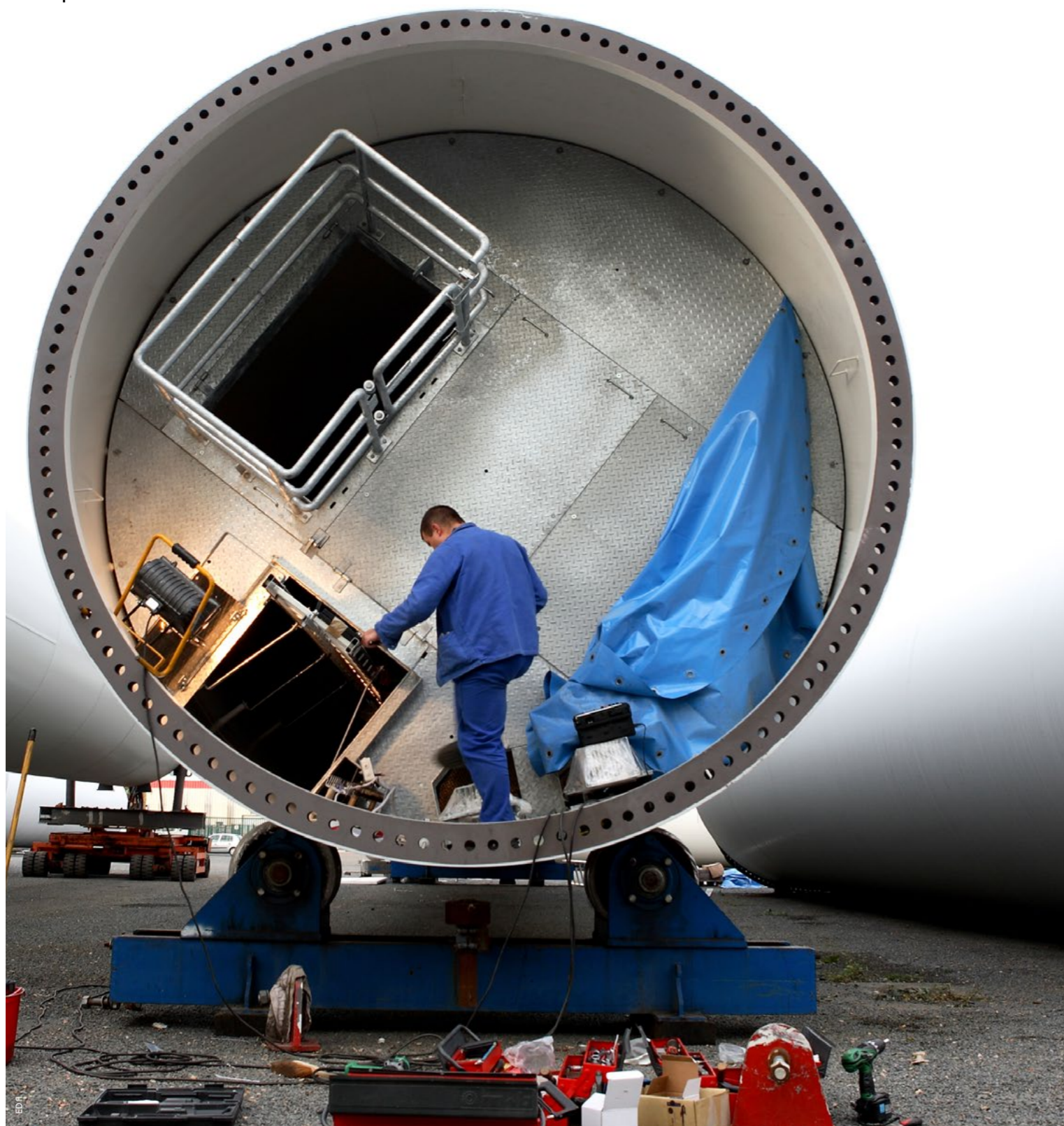
Installation of a lift on a wind turbine on the Harfleur enterprise zone.
